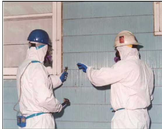
Pulling out nails
