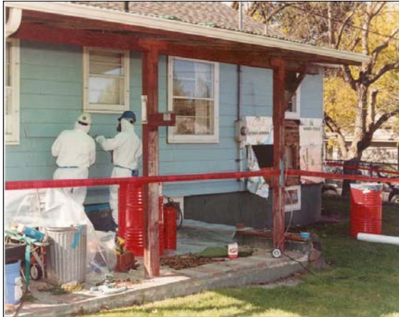
Prying to expose nail heads
