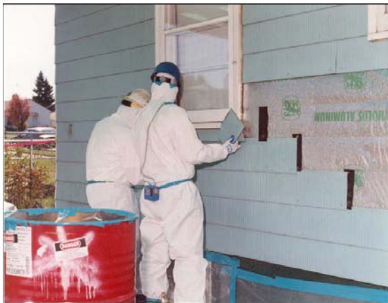
Removing siding
